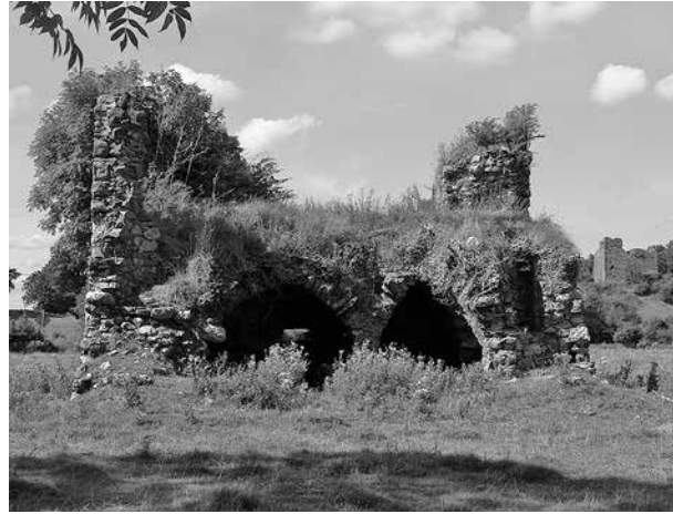
FIG. 14 Togher Castle, Doon, Co. Offaly: the base of a late fifteenth-century (?) tower-house, showing the twin-vaulted basement and the low surviving walls of the first-floor room above; a second tower-house is visible in the background on the right-hand-side ( photo by author )
