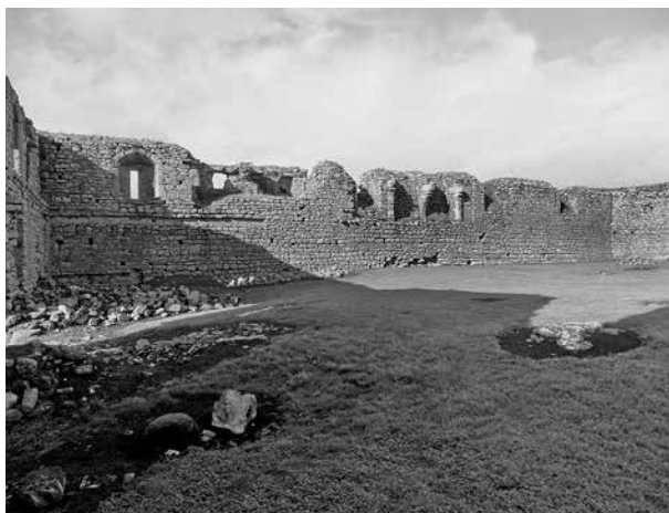
FIG. 8 The west side of the interior of Ballymoon Castle, Co. Carlow: the chamber was the room on the left, its precise position indicated by a horizontal chase for floor timbers, and the hall was the long room, heated by a double fireplace, that takes up the right-hand-side two-thirds of the wall ( photo by author )
