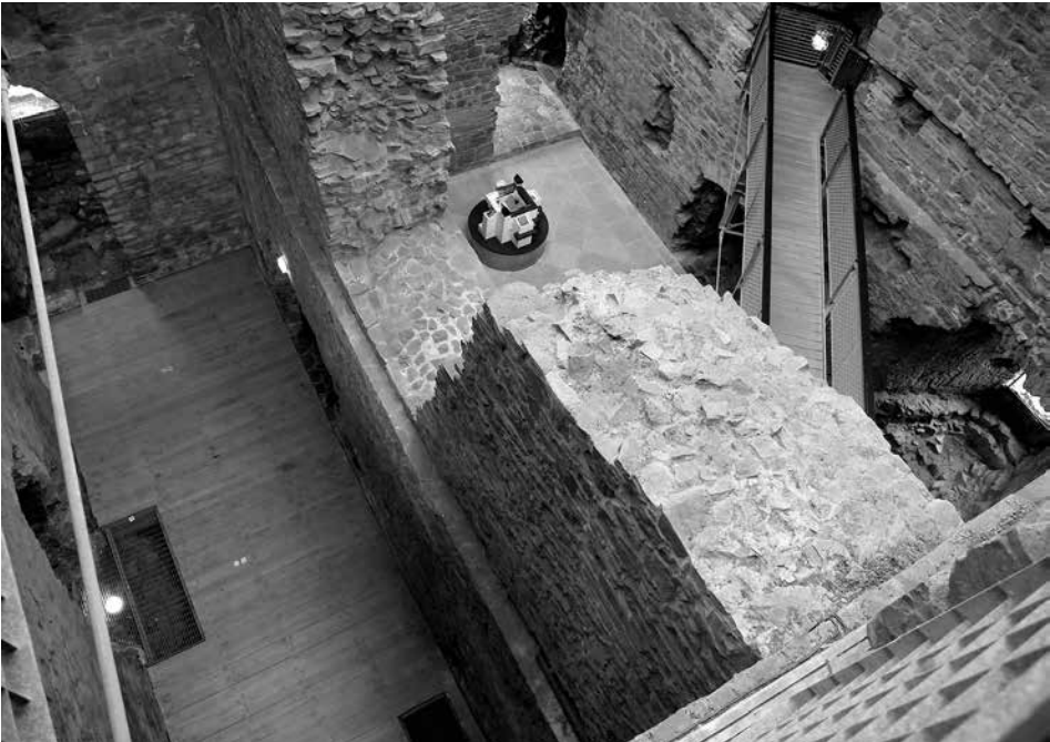
FIG. 2 The partitioned interior of Trim donjon, viewed from an upper storey level: the hall was on the right below the modern bridge, the chamber on the left (photo by author)
