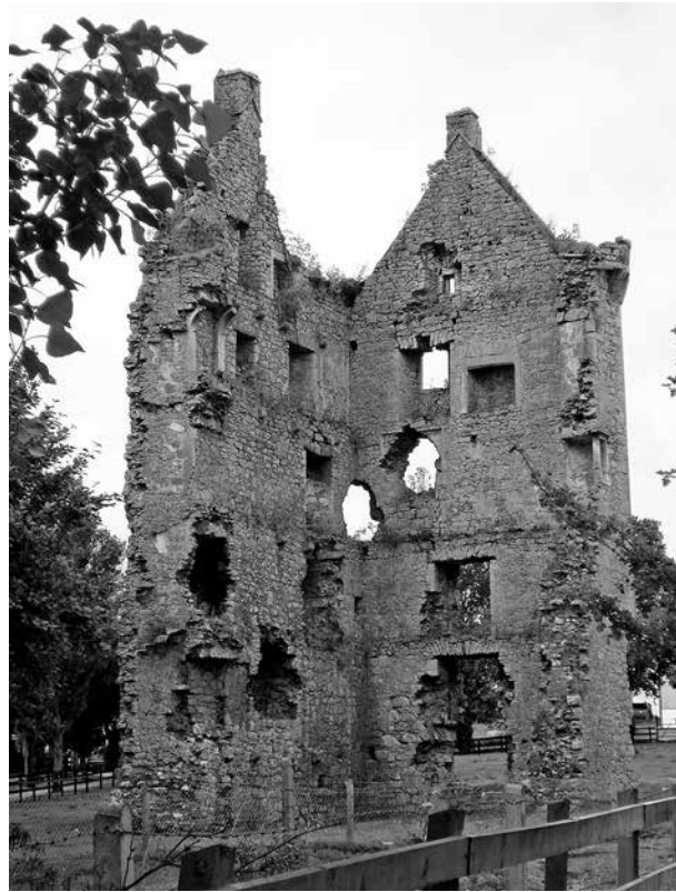
FIG. 19 Kilduff, Castle, Co. Limerick: a late sixteenth-century tower-house ( photo by author )
